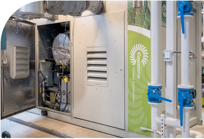
A C1000 microturbine at the VA Medical Center in Ann Arbor, Michigan provides electricity and steam to the 1.1-million-square-foot facility.
